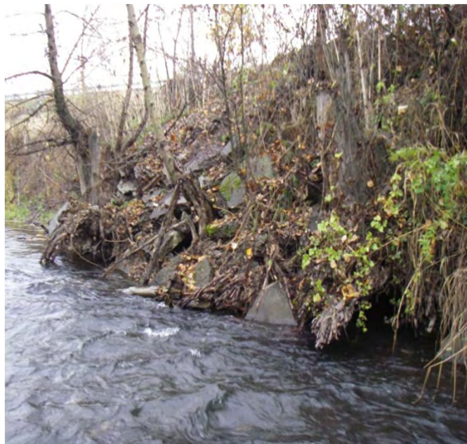
Photo 10. Broken concrete riprap end dumped along the right bank
