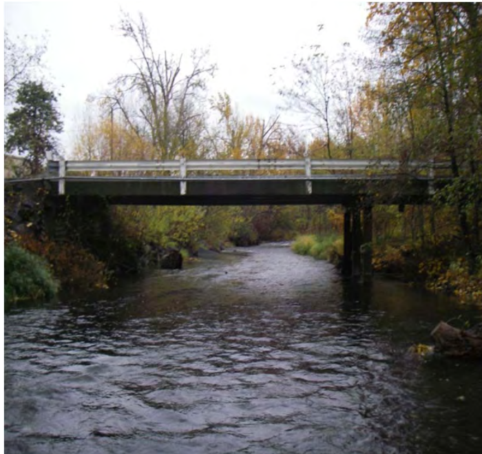
Photo 2. Upstream north fork bridge, looking upstream with one pier near left bank
