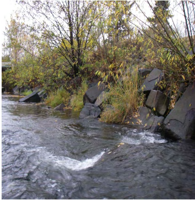
Photo 1. Right bank riprap protection, large basalt columns
