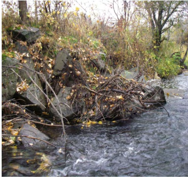
Photo 16. Riprap bank protection along the left bank, very localized
