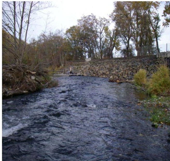
Photo 43. USACE's repaired section of levee along the right bank
