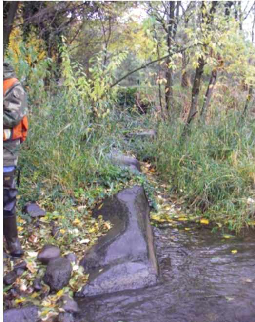
Photo 5. Rock barb along the left bank
