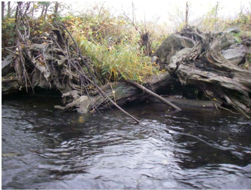
Photo 29B. Rootwads (5) with toe logs and rock ballast along the left bank
