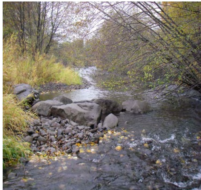
Photo 31. Rock barb along the left bank with large left side scour hole
