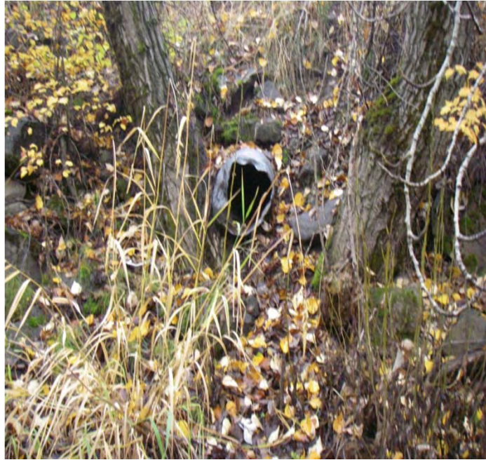
Photo 20. Drainage culvert entering the floodplain on the left bank upstream of the South Touchet Road bridge
