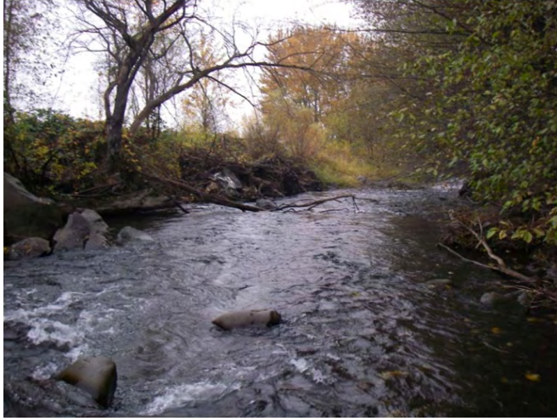
Photo 29A. Rootwads (5) with toe logs and rock ballast along the left bank
