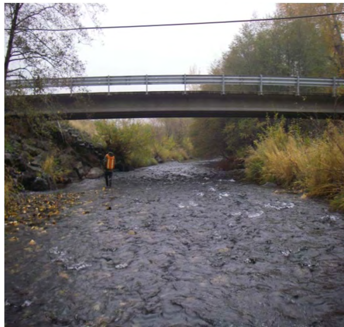
Photo 21. South Touchet Road bridge with abutment riprap on both banks
