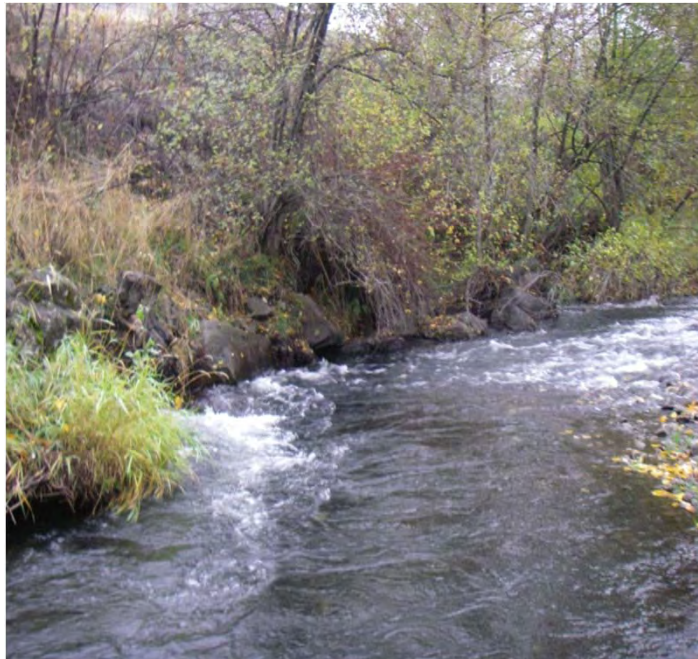
Photo 19. Rock and concrete riprap located along the right bank
