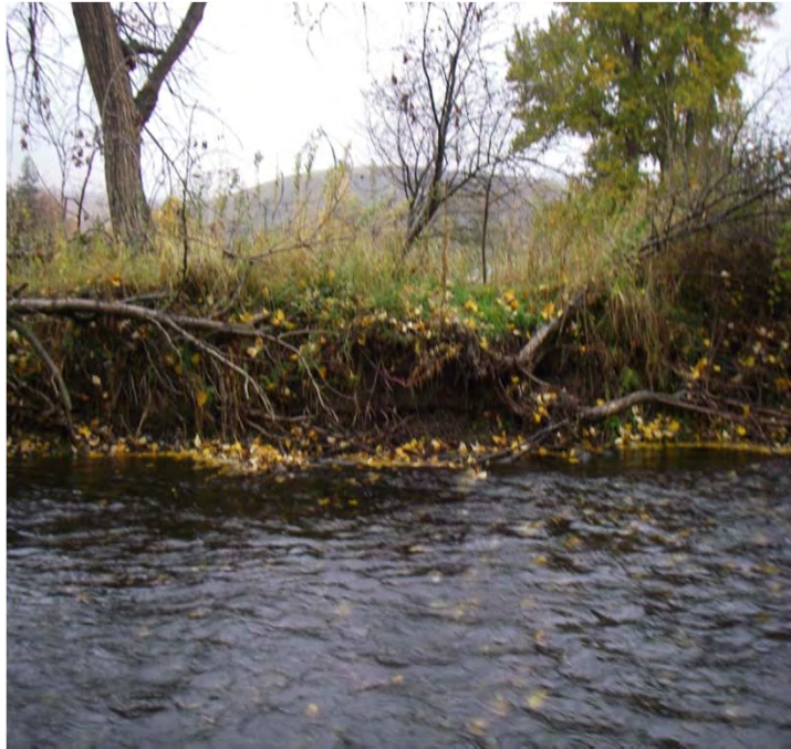
Photo 9. Cut bank and piping along roots along the left bank
