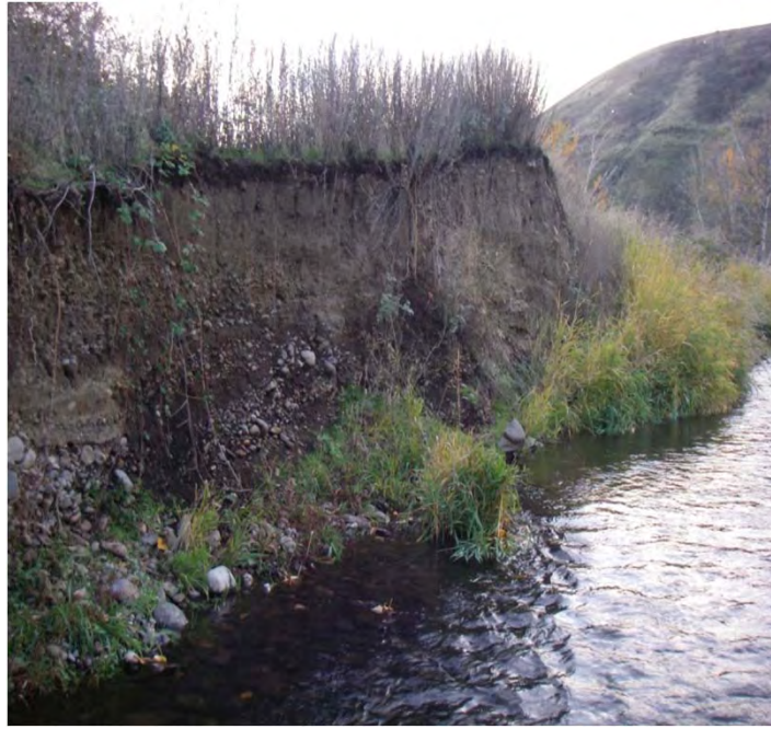
Photo 56. High cut bank along the right bank
