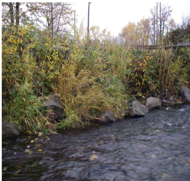
Photo 33. Point of diversion along the left bank
