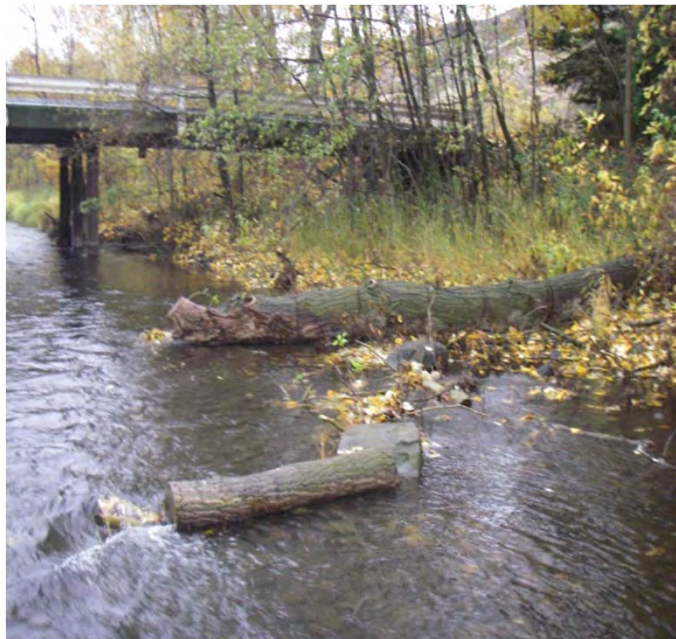
Photo 4. Cottonwood sweeper perpendicular to flow along left bank immediately downstream of bridge
