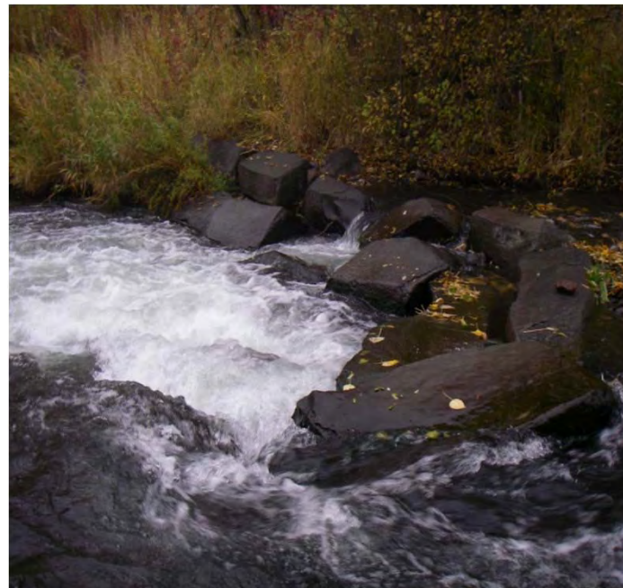
Photo 24B. Rock U-weir across the channel
