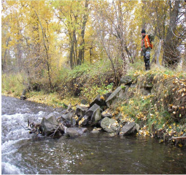
Photo 14. Rock barb along the left bank with some rock migration downstream
