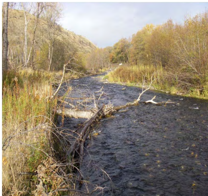
Photo 41. Small LWD elevated barb and channel log along the left bank
