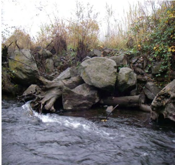
Photo 27. Distressed rootwads (6) with toe logs and rock ballast along the left bank
