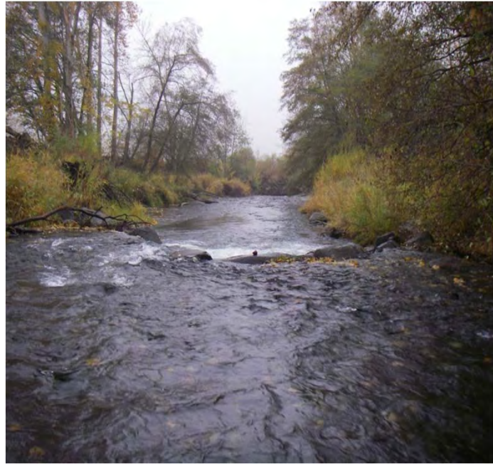
Photo 24A. Rock U-weir across the channel
