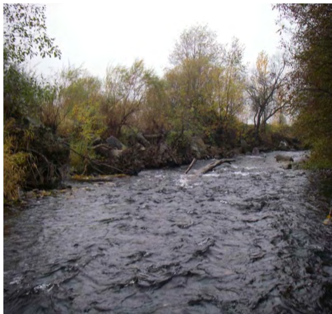
Photo 26. Rootwads (6) with toe logs and rock ballast along the left bank
