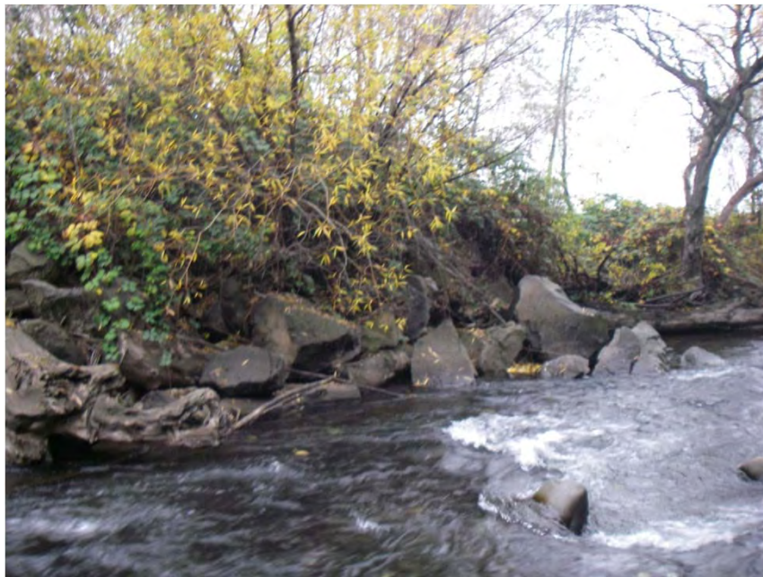
Photo 28. Short span of rock armoring along the left bank between LWD
