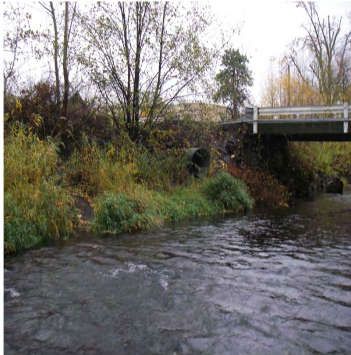
Photo 3. 24 inch drainage culvert along the right bank immediately downstream of bridge
