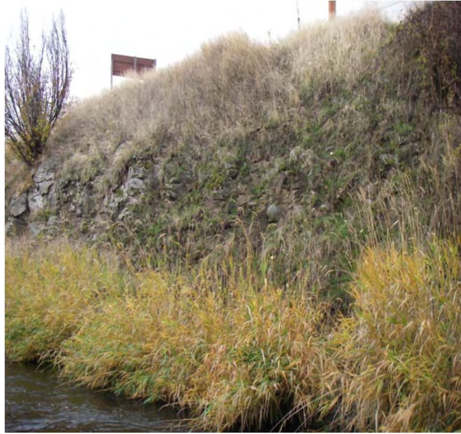
Photo 34. Weathered basalt along the right bank adjacent to the Touchet River Road
