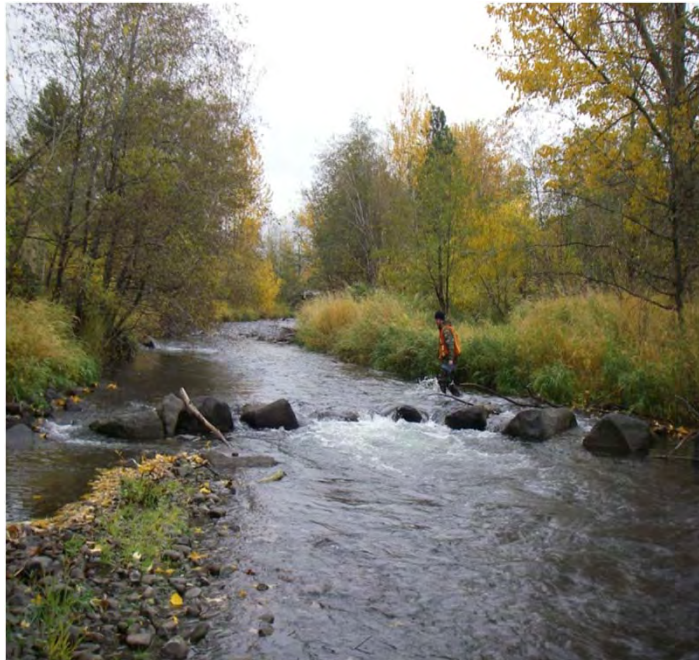
Photo 6. Channel spanning U-weir
