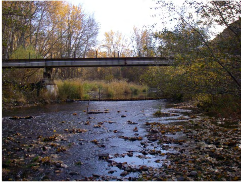
Photo 46. View upstream of private bridge along the South Fork Touchet near upstream project boundary
