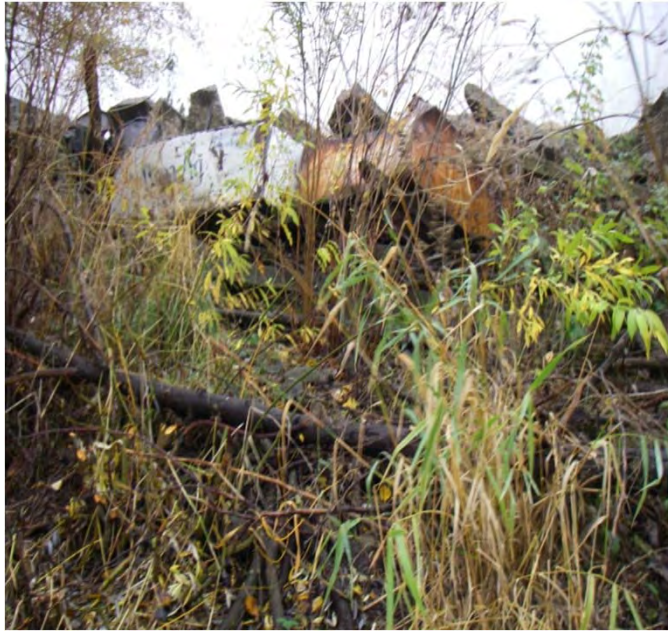
Photo 25. Concrete and metal revetment along the left bank
