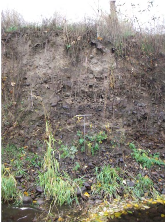
Photo 12. Erosion and actively cutting bank along the right bank at hardened bend
