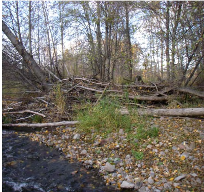
Photo 49. Overbank racking members and debris blocking along the right bank
