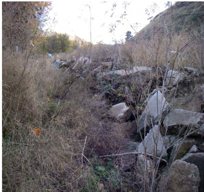
Photo 51. Concrete revetment along the left bank floodplain
