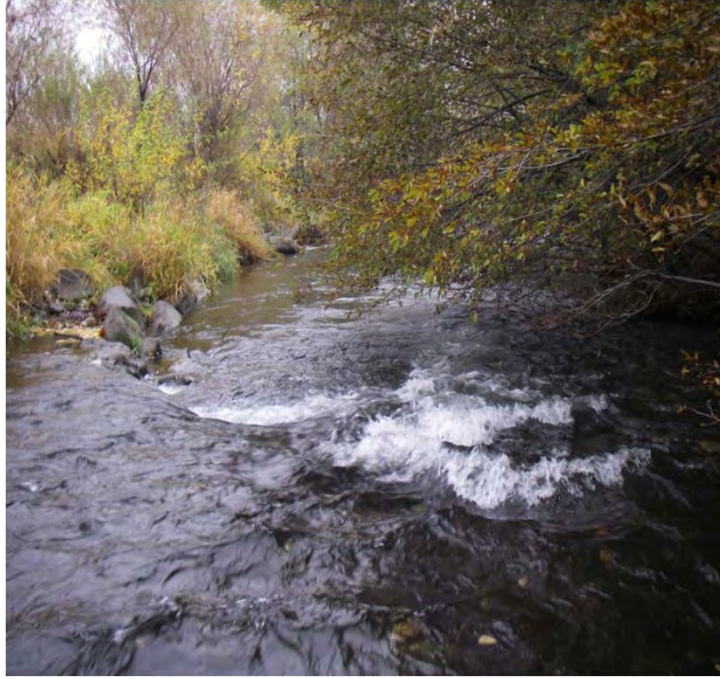
Photo 22. Rock barb on left bank
