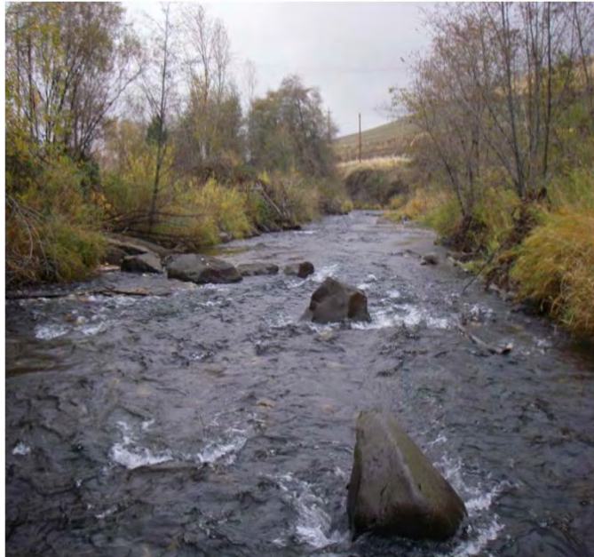
Photo 32. Short stretch of random boulders placed in channel
