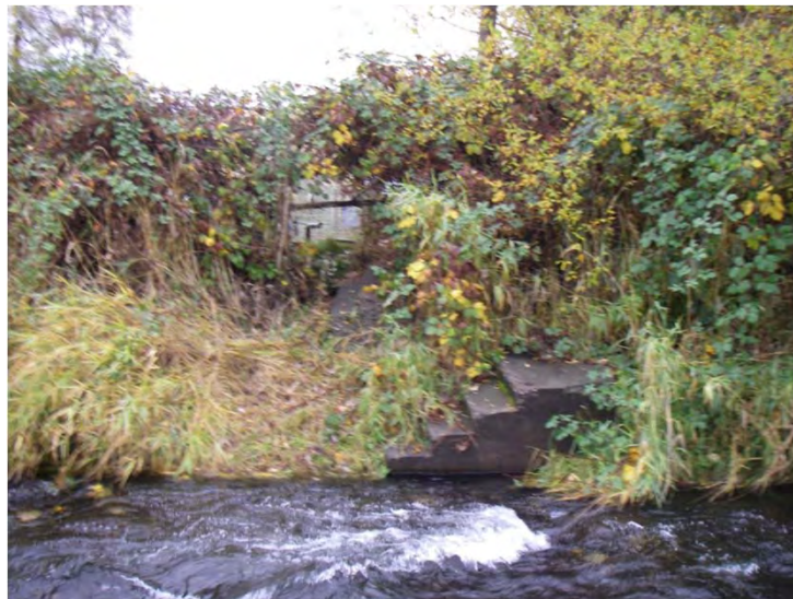
Photo 8. Concrete stair access along the right bank
